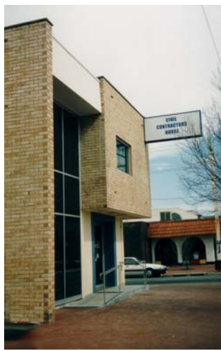
Earthmoving Contractors Association Head Office Fit Out, Woodville
